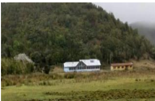
Current school near the project
